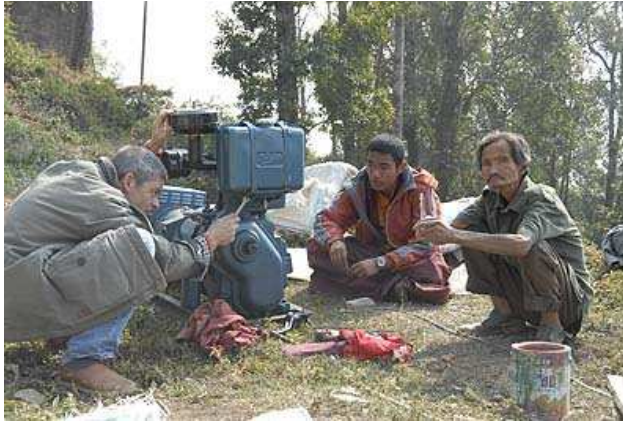
Peter installs the generator. Even in the first Puja-Night next power failure and the first kick on - from that moment on the monks call it "Mahakala-Generator".
